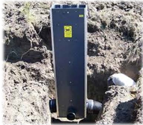
Water Control Structure
