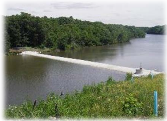
Low-flow/in-lake dam; Otter Lake, Illinois
