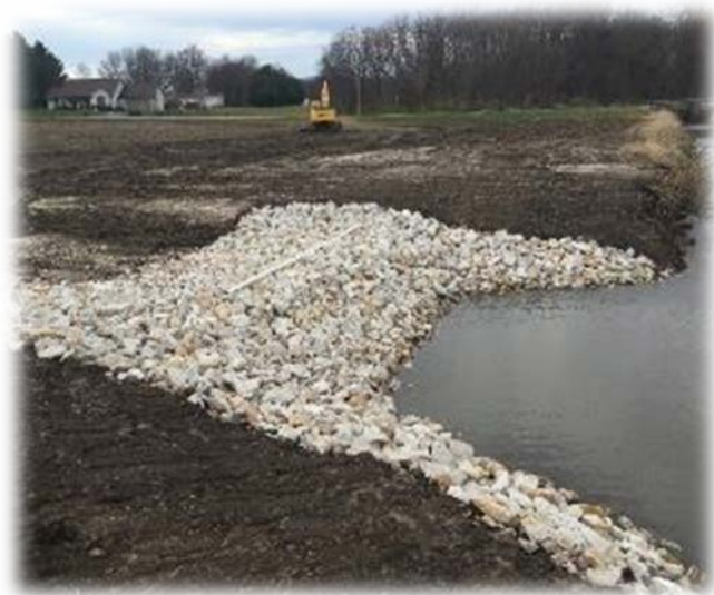
Grade Control Structure
