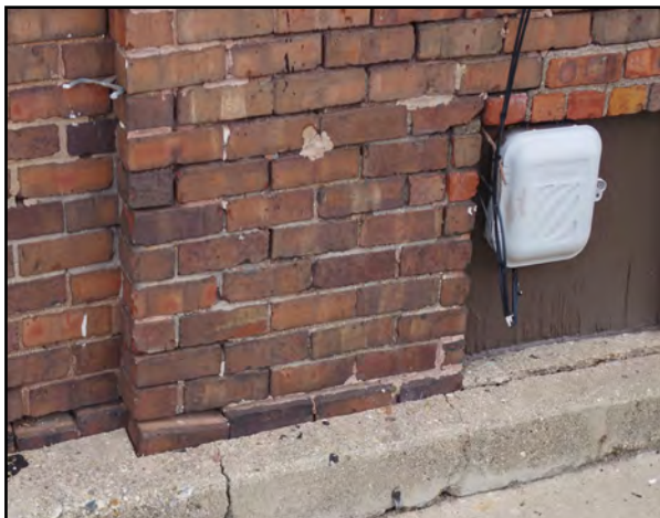
Left & Right: The mixed use building is in need of tuck-pointing.
