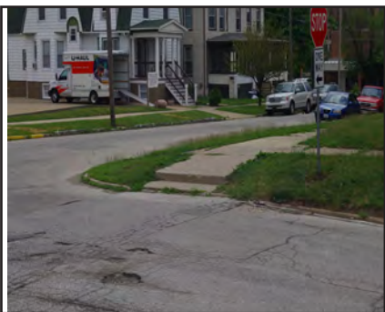
Below: The pavement and curbs are deteriorated at the intersection of Gridley and Jefferson.
