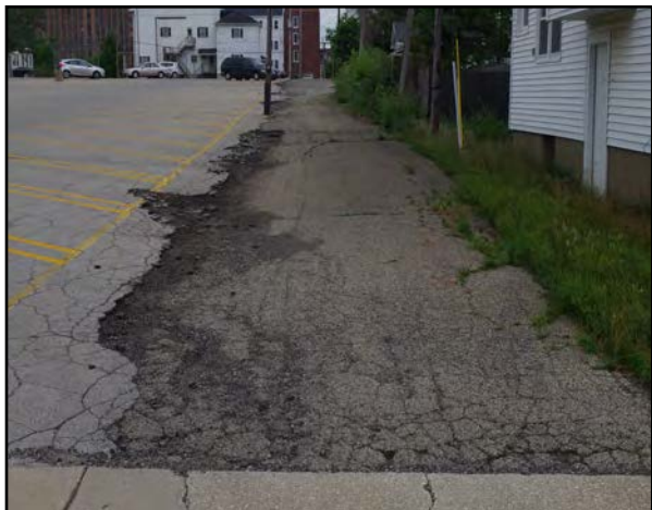
Left & Right: The edge of the pavement at 402 East Jefferson Street is crumbling and deteriorated.
