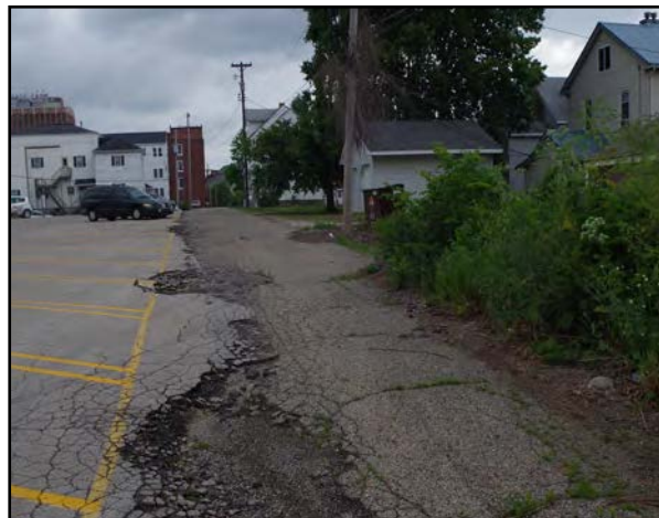
Left & Right: The edge of the pavement at 402 East Jefferson Street is crumbling and deteriorated.
