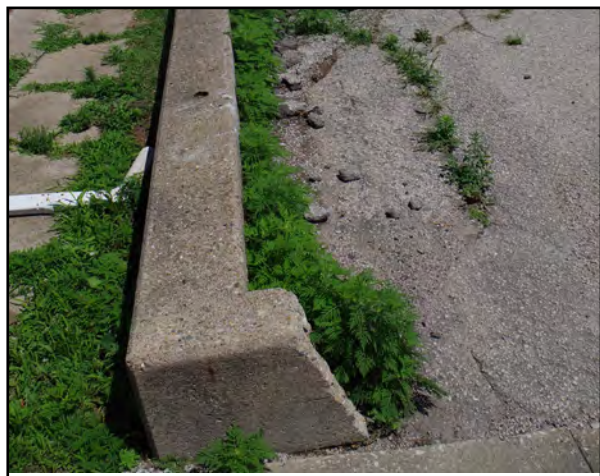
Left: The retaining wall on the north side of 500 East Jefferson is leaning.
