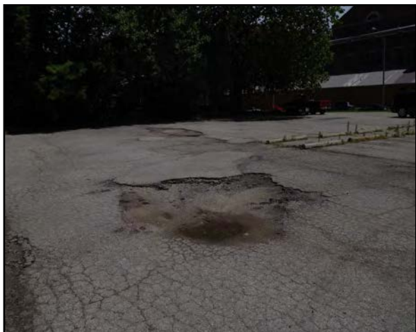
Left: The parking lot at 500 East Jefferson is deteriorated and contains large potholes.
