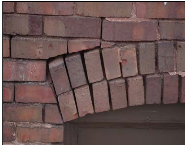
Left & Right: The mixed use building is in need of tuck-pointing.
