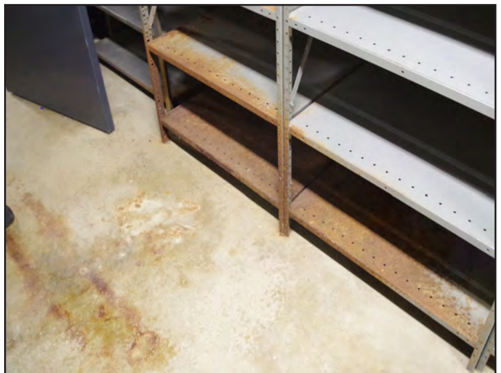
The metal shelving in the basement has rusted as a result of the moisture infiltration.
